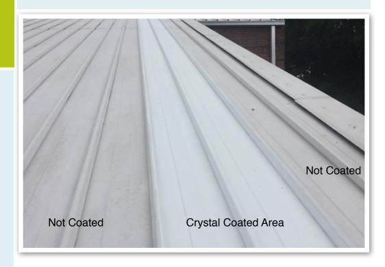
An application trial of Crystal clear insulating and mold & UV resistant roof coating was done on a white metal roof on a school in Florida in order to prove the 'stay clean' and mold resistant capabilities of the coating.
