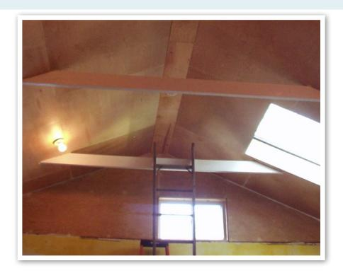
"I recently re-roofed my bungalow style house and added a skylight, ridge vents and soffit vents for a good ventilating air flow from the eaves to the peak. Inside I removed the old ceiling and attic insulation opening up part of the house with a "cathedral" ceiling and making a sleeping/ storage loft over the rest. I sheathed the inside of the roof rafters with furniture grade birch plywood and sealed this with translucent HomeProtect™.
