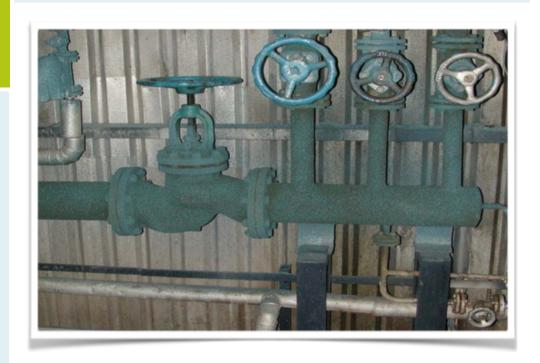
Heat Shield™ High Heat was used as a primer beneath a 2.5 to 3mm application of Heat Shield™ EPX-H2O.
