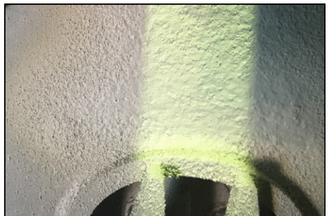
Boiler end cap with EPX-H2O coated area
