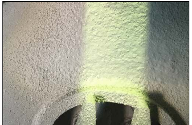
Boiler end cap with EPX-H2O coated area
