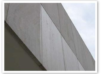
The entire wall was cleaned and the three lower tiles were coated with 2 coats of Energy Protect<sup>™</sup> coating. After 1-year this photo was taken. The coated area was still free of any mold growth, while mold had returned as usual to the untreated marble areas.
