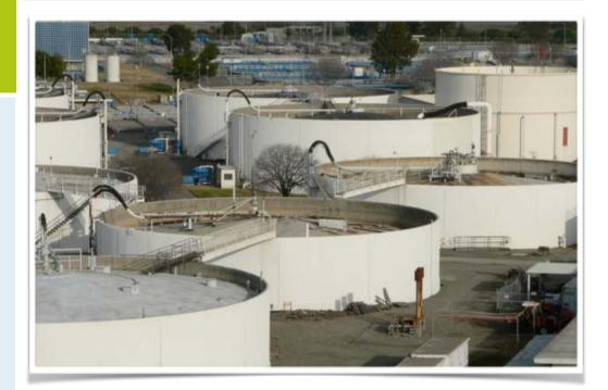
The city of San Jose California was looking for a cost effective way to insulate and protect their exterior of their concrete waste water digester tanks. They recapture the heat from the digester process and use that to power other systems, so insulating the tank means more energy captured for reuse.
