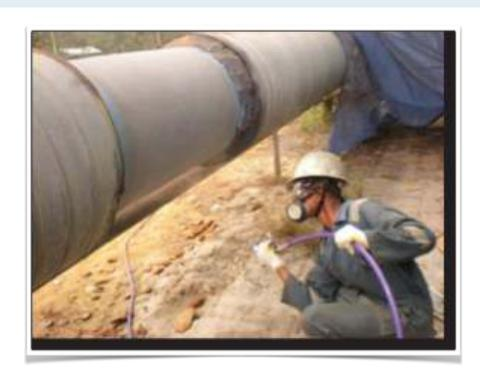
large client for PT Nukote Indonesia needed to reduce the surface temperature of a hot water pipeline from the variable 74-95 deg C surface temp to 65 deg C or lower. They also wanted corrosion resistance to protect the pipeline and increase the lifespan. Their prior experience with corrosion under insulation (CUI) and the short lifespan of traditional insulations meant they needed a new technology solution.
