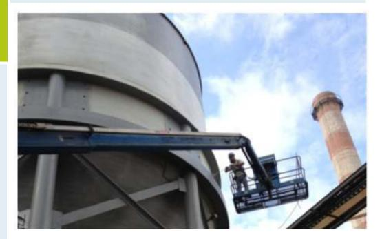
Large paper manufacturer, Weyerhaeuser, was looking for a way to effectively insulate an outdoor liquor tank while also reducing surface temperature and providing protection from corrosion and weathering.
