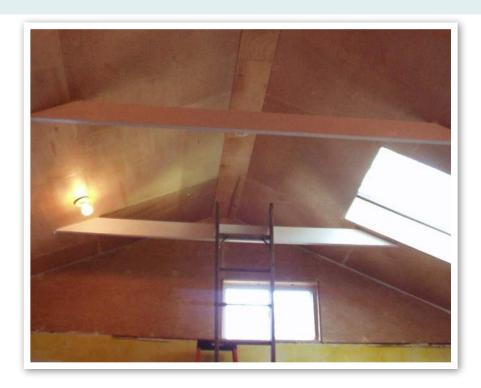
"I recently re-roofed my bungalow style house and added a skylight, ridge vents and soffit vents for a good ventilating air flow from the eaves to the peak. Inside I removed the old ceiling and attic insulation opening up part of the house with a "cathedral" ceiling and making a sleeping/ storage loft over the rest. I sheathed the inside of the roof rafters with furniture grade birch plywood and sealed this with translucent HomeProtect™.
