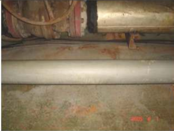
Final aspect without primer. Middle section
