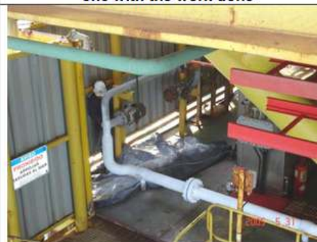
First section during work.
