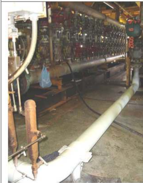
Last trace of the pipeline before pumping.
