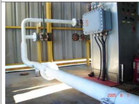
First section. Work done
