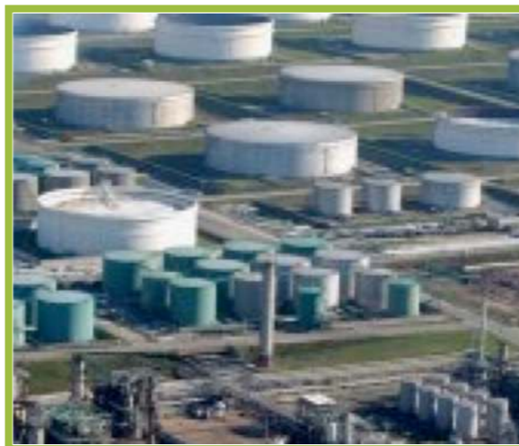
Pipeline & Storage Tank Insulation Galp Energia Portugal
