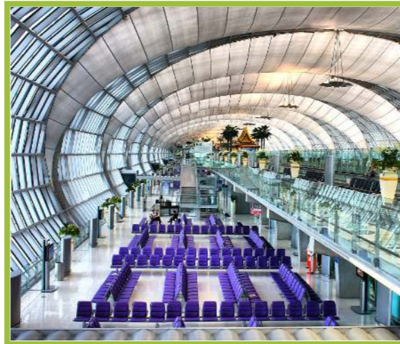
Energy Savings & Sustainability International Airport Bangkok, Thailand
