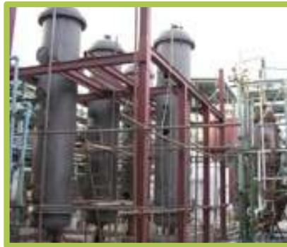
Brine Reactor Column Insulation Chemical Manufacturer Middle East
