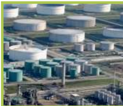
Pipeline & Storage Tank Insulation Galp Energia Portugal
