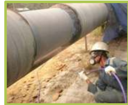
Insulation & Corrosion Control Hot Water Pipeline Indonesia
